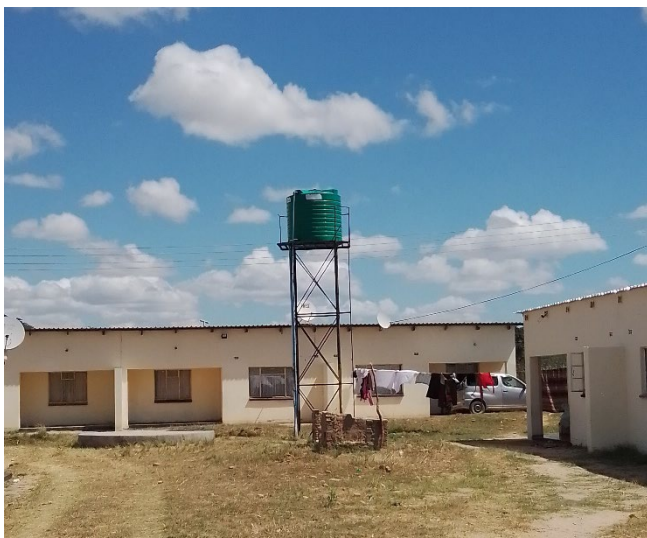
New tanks to equalize water supply through pressure pumps
