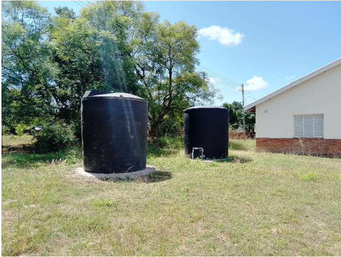
Optimization of existing tanks after the installation of a new borehole with prolific water supply and connected 24/7 to the hospital generator through an overhead line.
