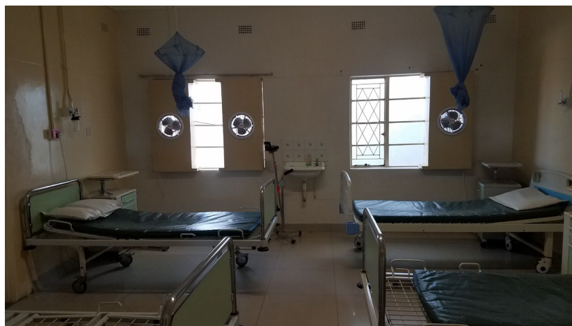
The completed renovation ( above ). Below , images of the COVID19 isolation ward with forced ventilation realized to guarantee > 12 air-room changes/hour.
