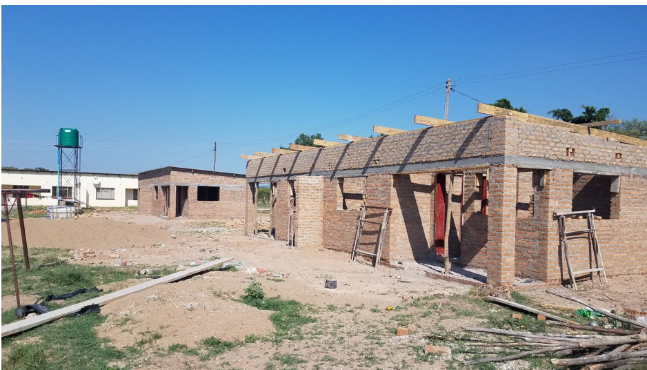
Two houses for staff under construction within the hospital premises
