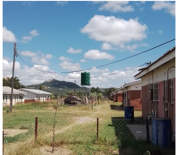
Optimization of existing tanks after the installation of a new borehole with prolific water supply and connected 24/7 to the hospital generator through an overhead line.
